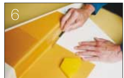
6 Repair of imperfections in joints by the use of a wax infill.
