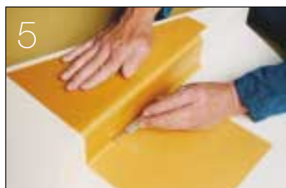
5 Consolidation of corners using filleting tools.
